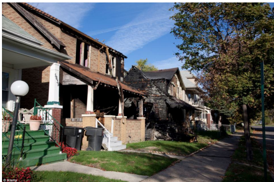
Figure 5-Deteriorating Detroit neighborhood-Daily Mail-Photo Marchand-Meffre
